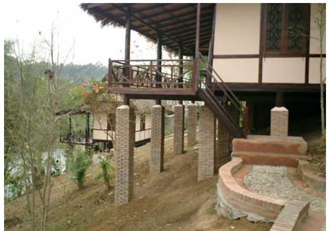
Ecolodge construction on a slope
