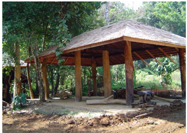
Carefully cleared land
