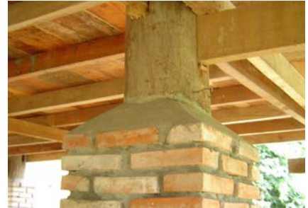
Brick wrap around foundation
