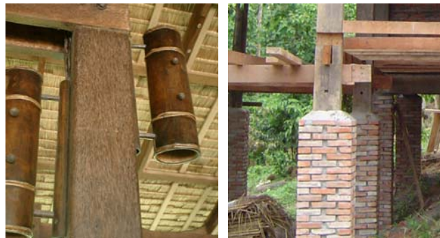
Examples of exposed wooden pillar supports
