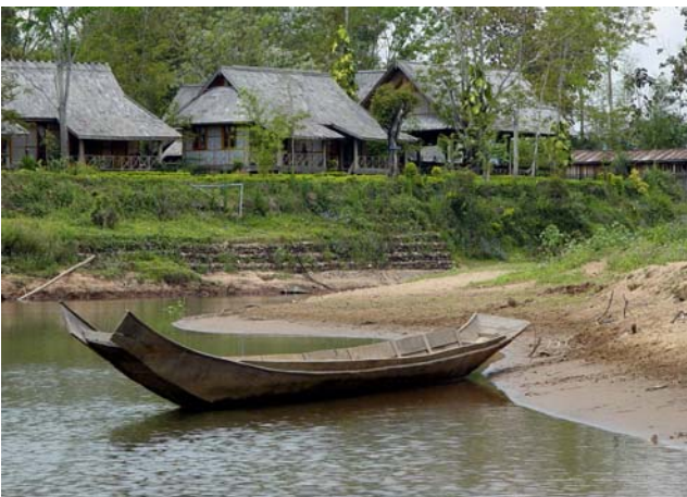
Erosion of a riverbank
