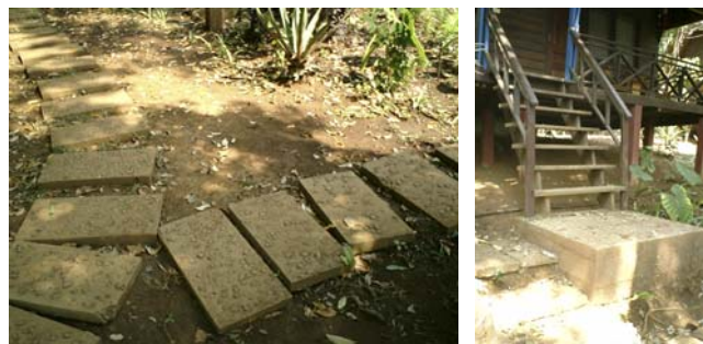
Your guests can be easily injured on uneven walkways or stairs that are too steep
