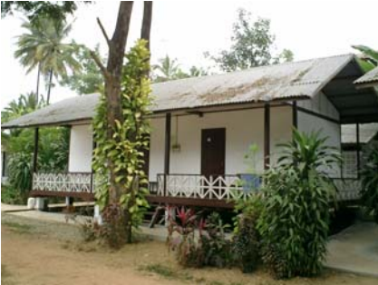
Tin roofs are hot and noisy
